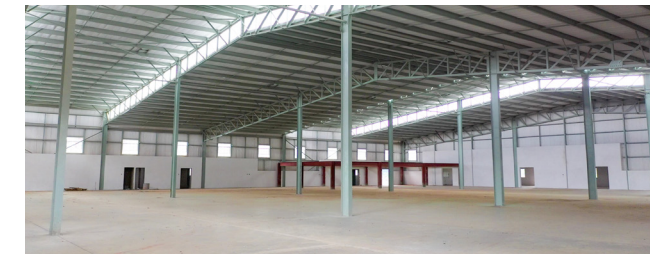
Belo Industrial Park, Buthe.
