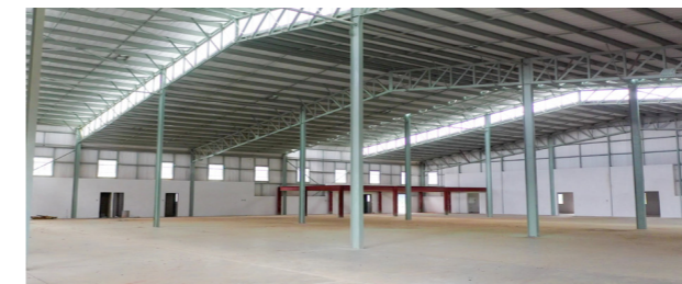
Belo Industrial Park, Buthe.
