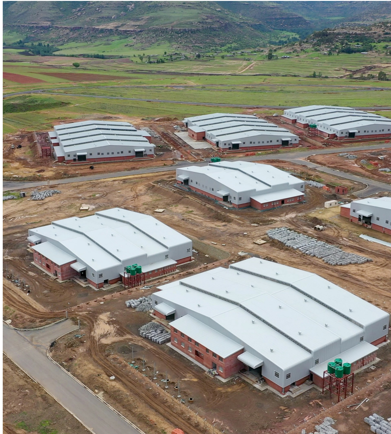
Belo Industrial Park, Buthe.
