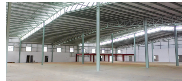
Belo Industrial Park, Buthe.
